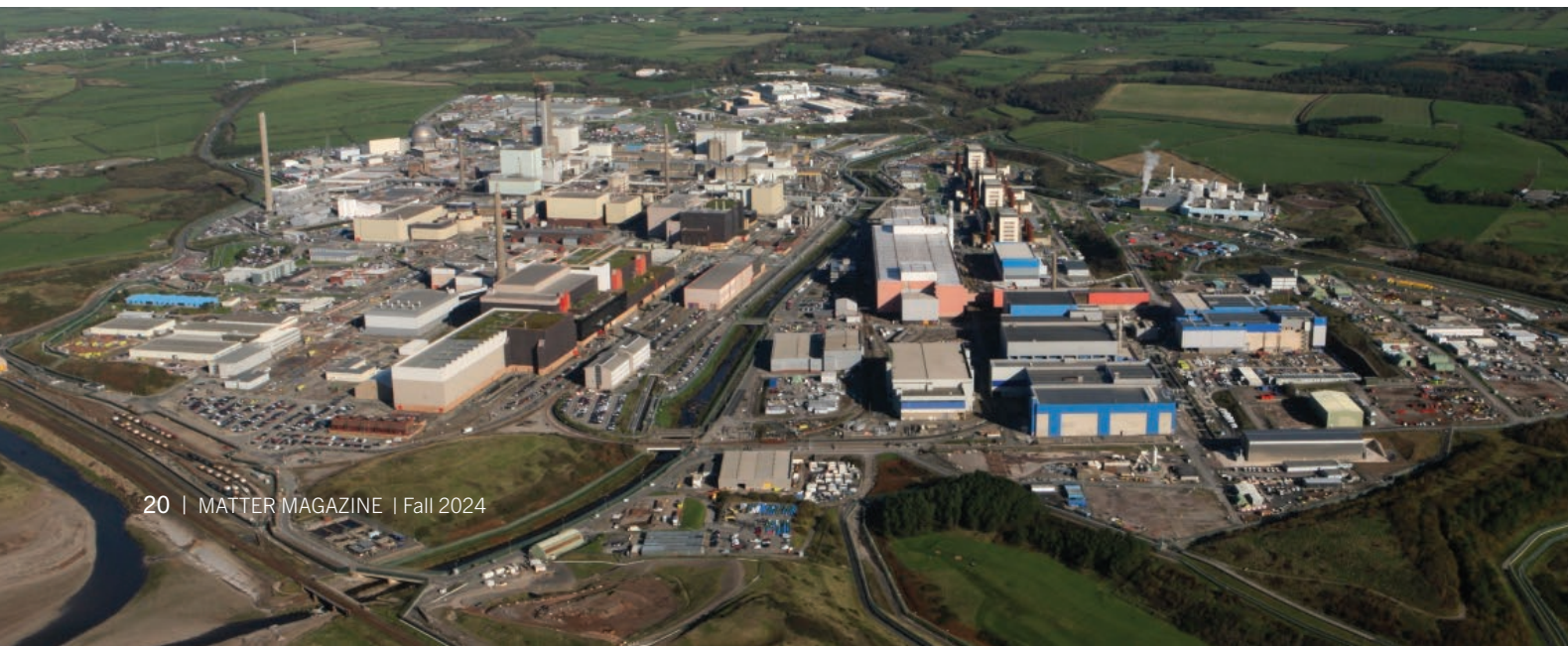
Aerial image of Sellafield Ltd. located in Cumbria, England, a new location where ALTEMIS is being installed. (Sellafield Ltd. Photo)
